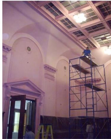
*Left: Workers begin preparing the Memorial Room for restoration. The work includes repainting the walls and ceiling, polishing and lacquering the brass railings, cleaning and polishing the Terrazzo floors, cleaning the hard surface artifacts and inventorying and cataloguing all the items in the room. Alumni volunteers have donated many hundreds of hours to date.*
