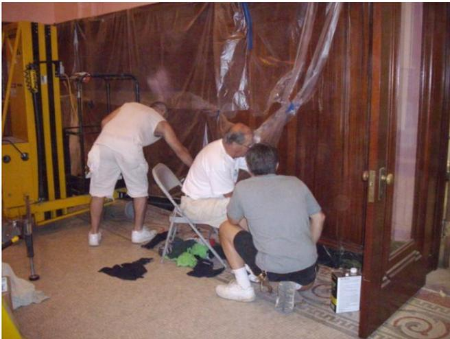
Above: Contractors and TPS Facilities Manager, Bill Birch, inspect mahogany wall restoration efforts. This section of the wall was damaged during the 2006 water leak. Experts have been able to restore the wall to its 1907 condition.
